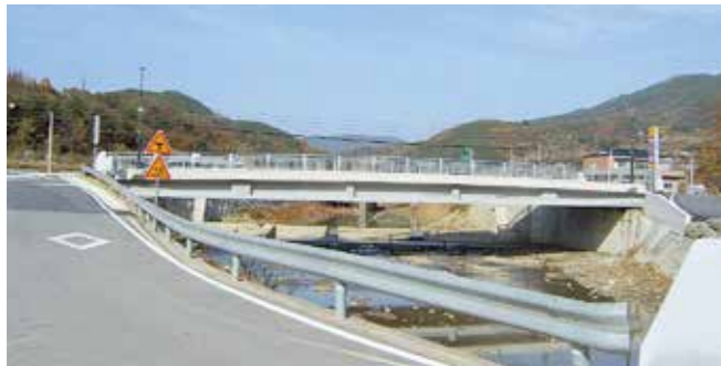
CHA HANG BRIDGE (韓国:SPC合成桁橋)
